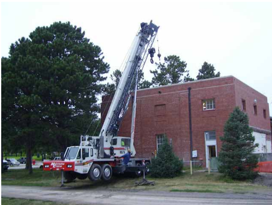
Workers install a new boiler for the biomass project.
