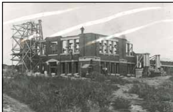
Construction of Ag Hall, 1912.
