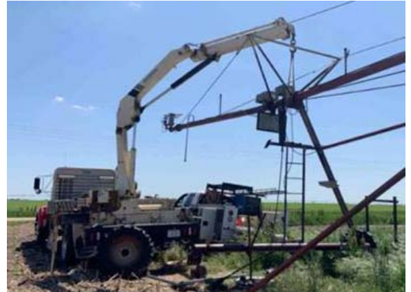
Jarrod Tuttle applies irrigation technology skills in replacing a center pivot tower leg at his summer internship. (Courtesy photo)
