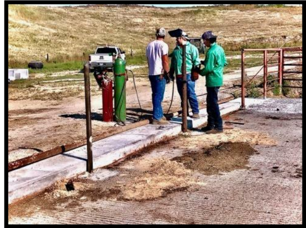
Advanced welding course students have been rebuilding steel pens at the NCTA feedlot. (Stehlik / NCTA photos)
